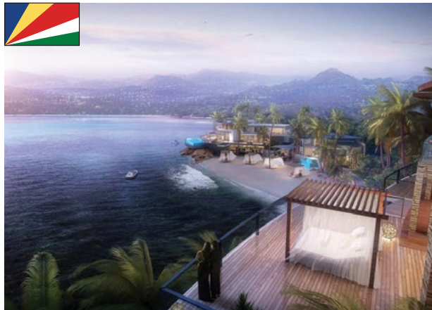
Mango House Project
