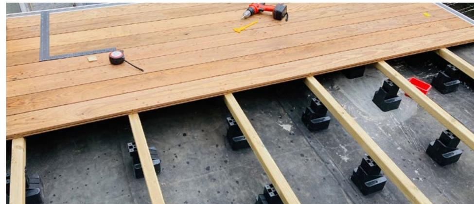
RAPTOR Series - height range from **3/5** to **9 2/3** inch (from 15 to 245 mm)
